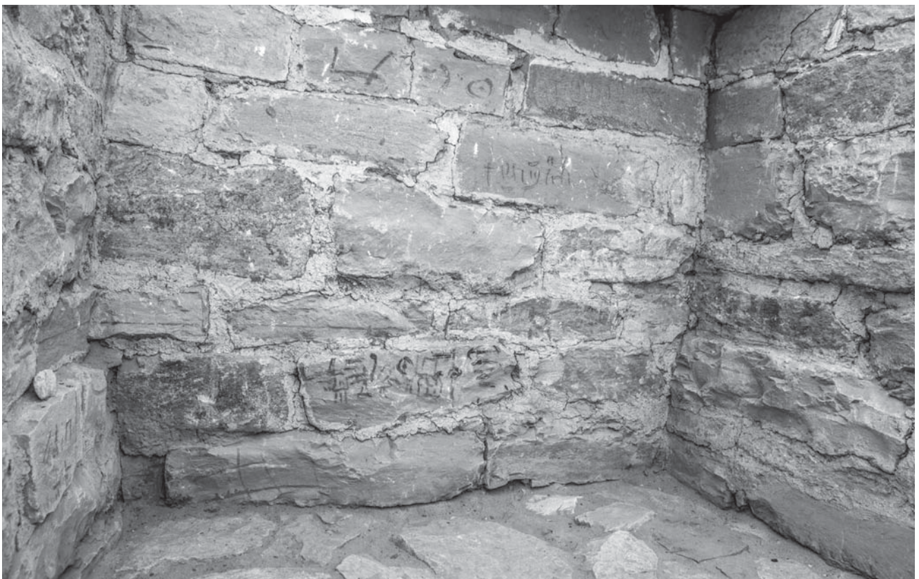
Fig. 6 Masons' inscriptions (including the title and name of the tomb owner) and construction lines on the western wall of the burial chamber (photo J. Krejčí)
