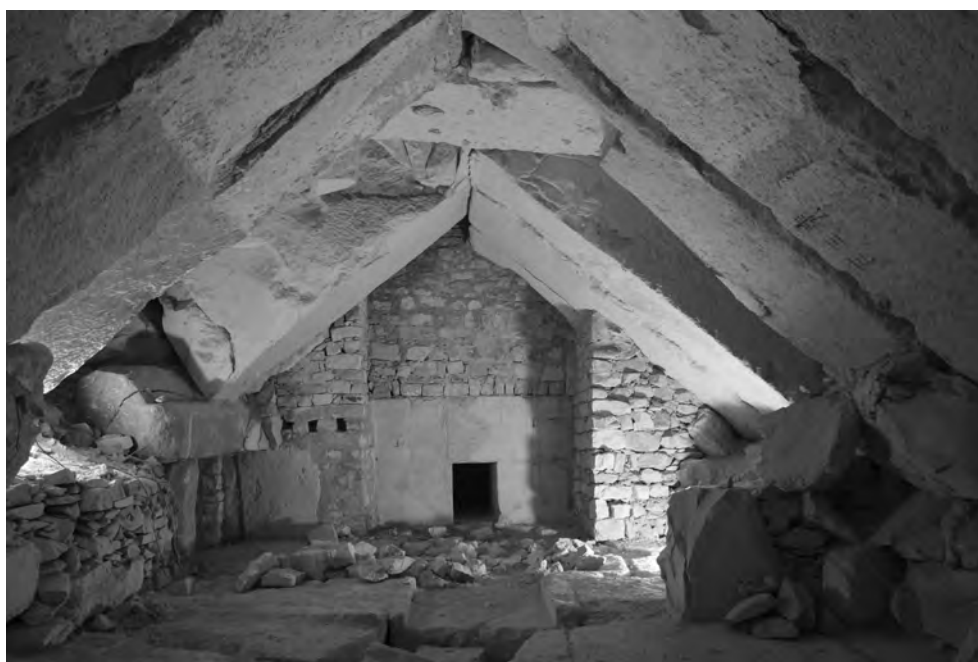
Fig. 18 The consolidated east wall of the antechamber of Djedkare's pyramid (photo H. Vymazalová)
